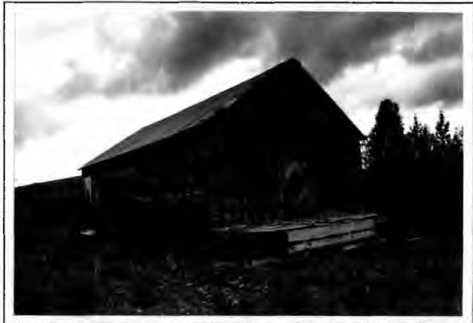
Figure 38. The Turner/Donnelley Hardware Building, 1993, The view is looking northwest.
